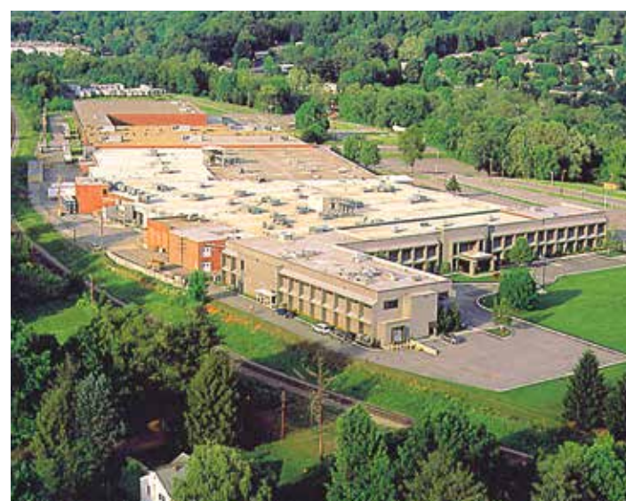
AERUS MANUFACTURING PLANT | BRISTOL, VA
